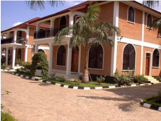
Figure 8. Building with Hydraform Dry Stacked Interlocking Blocks
