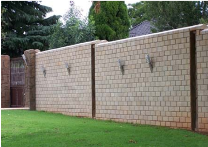
Figure 10. Boundary wall with Interlocking Blocks
