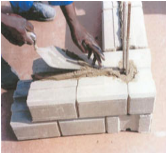
Figure 9. Vertical Steel in Masonry
